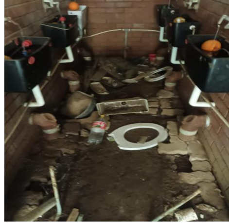
State of the toilets before the upgrade
